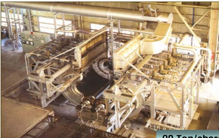
90 Ton/charge Roll rapid heating furnace for roll surface
